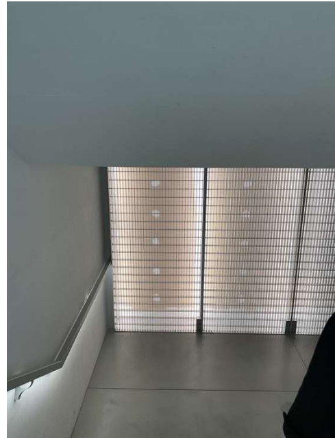
Fig. 13 – Rough aesthetics on the stairs of the Tower.
