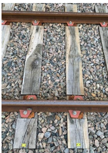
Fig. 1 – Ballast, traverses, rail (Biars-Bretenoux).
