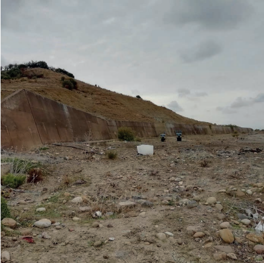
Figure 4. Left bank secondary levee (Picture by anonymous)
