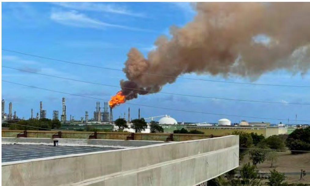
Figure 6. Malfunctioning flare at Limetree Refinery emitted smoke and droplets of crude oil in spring 2021 (photo submitted by resident to Community Impact Survey project).
