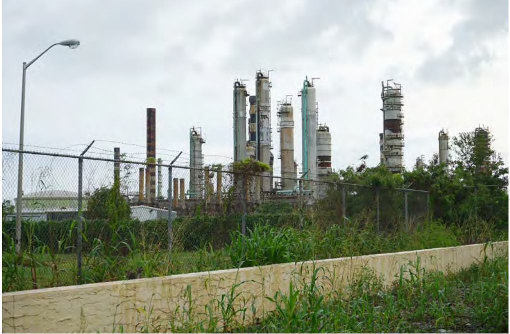
Figure 4. Damage to Hess/Hovensa/Limetree Refinery after Hurricane Maria (by Author).
