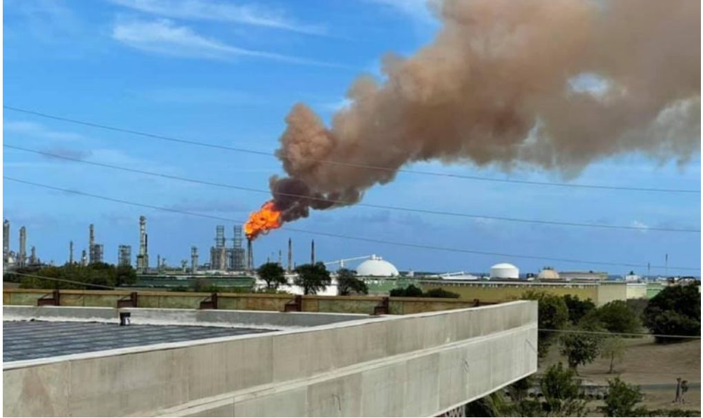
Figure 6. Malfunctioning flare at Limetree Refinery emitted smoke and droplets of crude oil in spring 2021 (photo submitted by resident to Community Impact Survey project).
